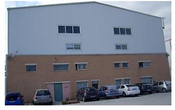
Fig. 1: Concrete-steel frame (Hybrid building) https://taxonomy.openquake.org/index.php/terms/hybrid-lateralload-resisting-system-lh
